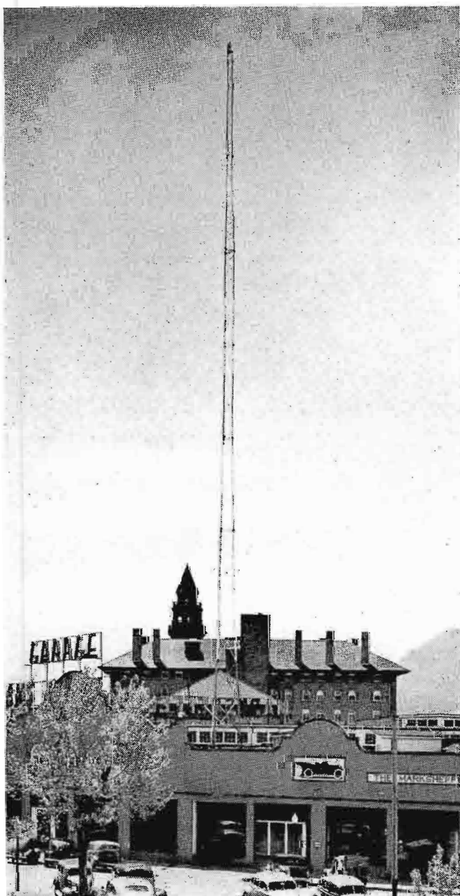
FIG. 1. Tower insulators of the KRDO antenna are located 25 feet above the ground level of a one-story garage.
