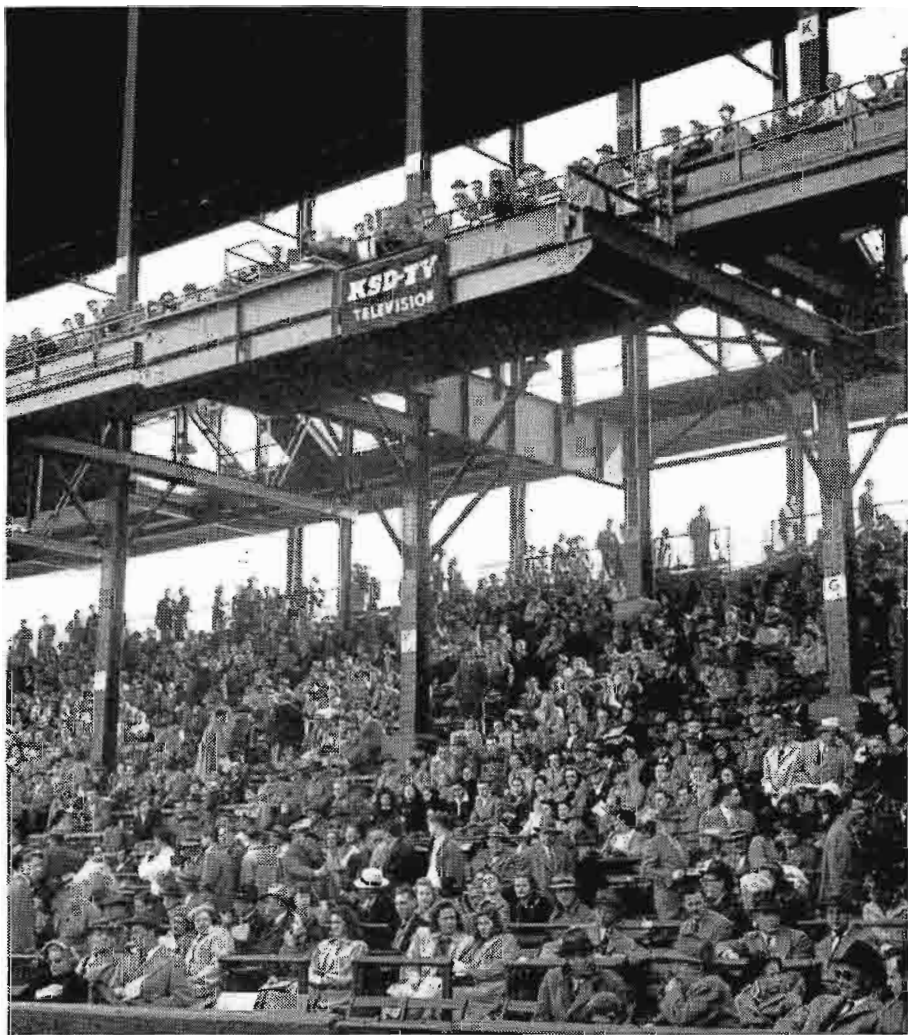
This shows how the special booth was built out from the second tier to provide KSD-TV with its vantage point. All cables and audio facilities are installed permanently to facilitate setup.
