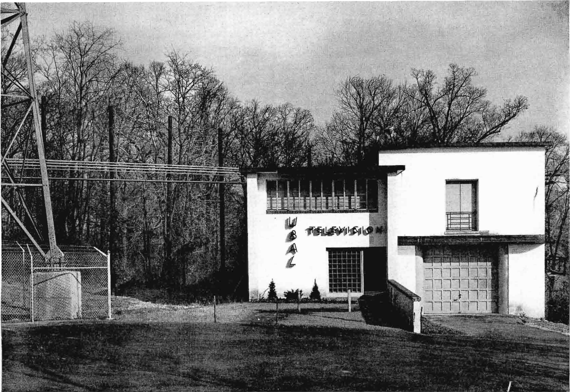
FIG. 12. The modern transmitter building contains a garage for Mobile Unit, workshop, office, kitchen, and the transmitter room. Feed lines, supported by several sturdy poles, are routed up the tower (left) to the 6-section Superturnstile.
