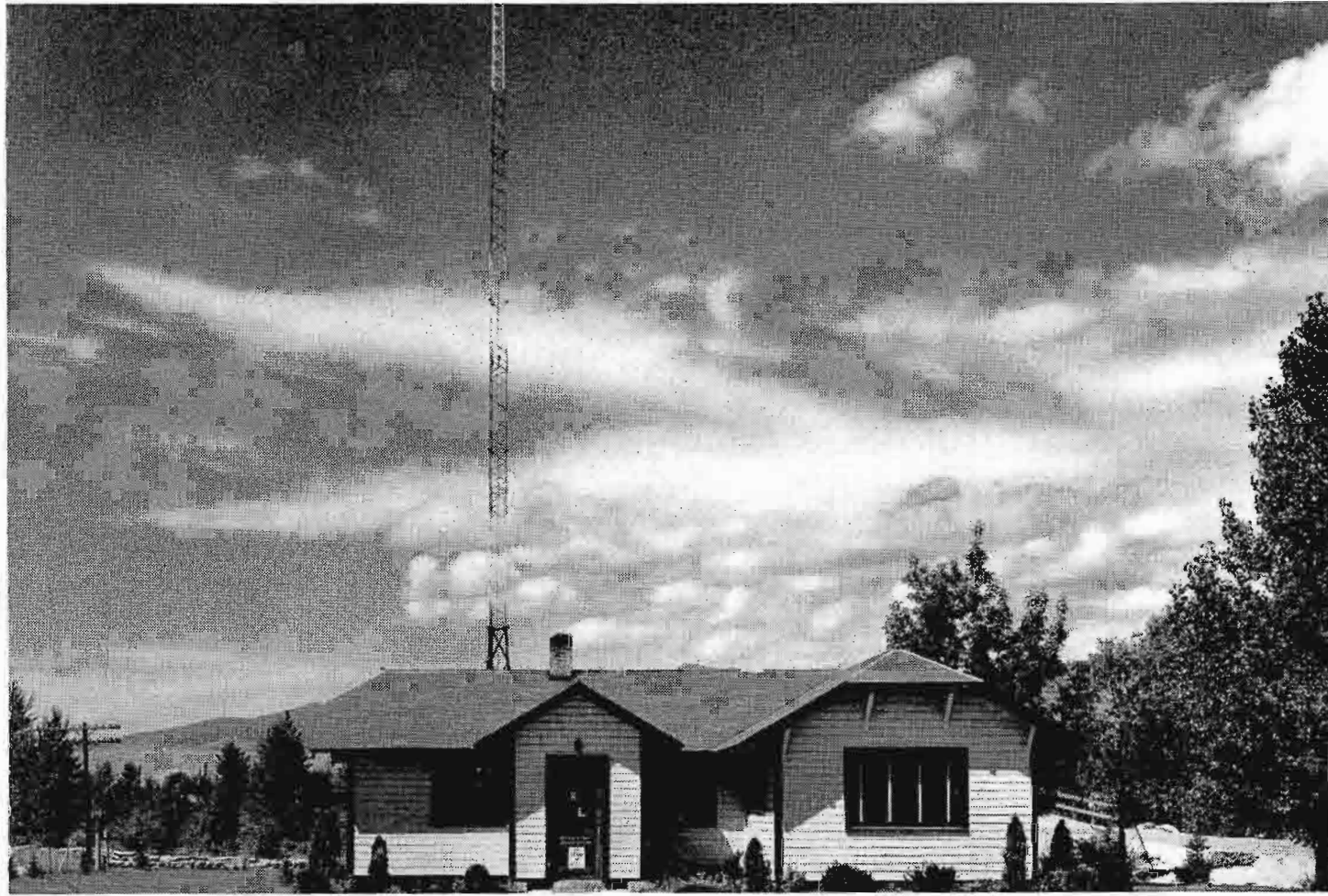
FIG. 1. Shown above is the transmitter building of KXLL which is situated about 200 feet from a river. The antenna tower shown at rear of the building is located at river's edge with half its ground system buried under water.
